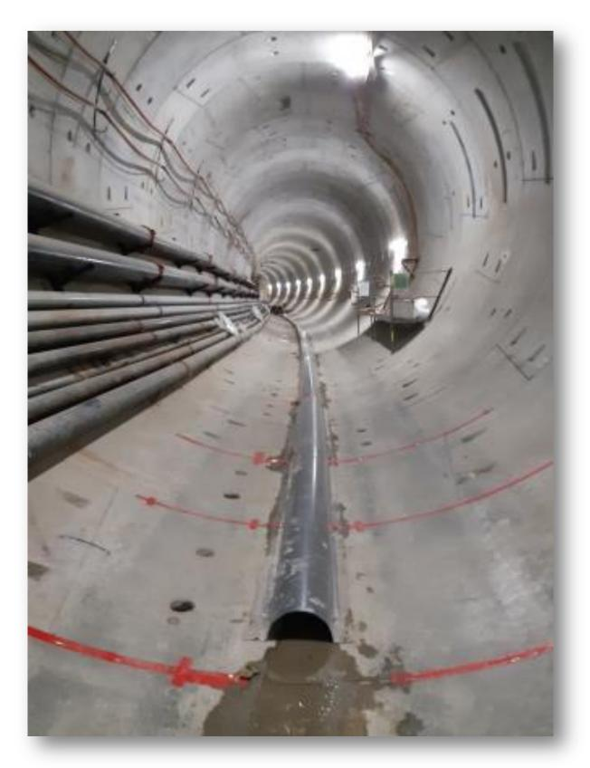
300mm Invert Drain (TP890) installed in 6m lengths for the Forrestfield Airport Link Tunnel in WA (2020)
