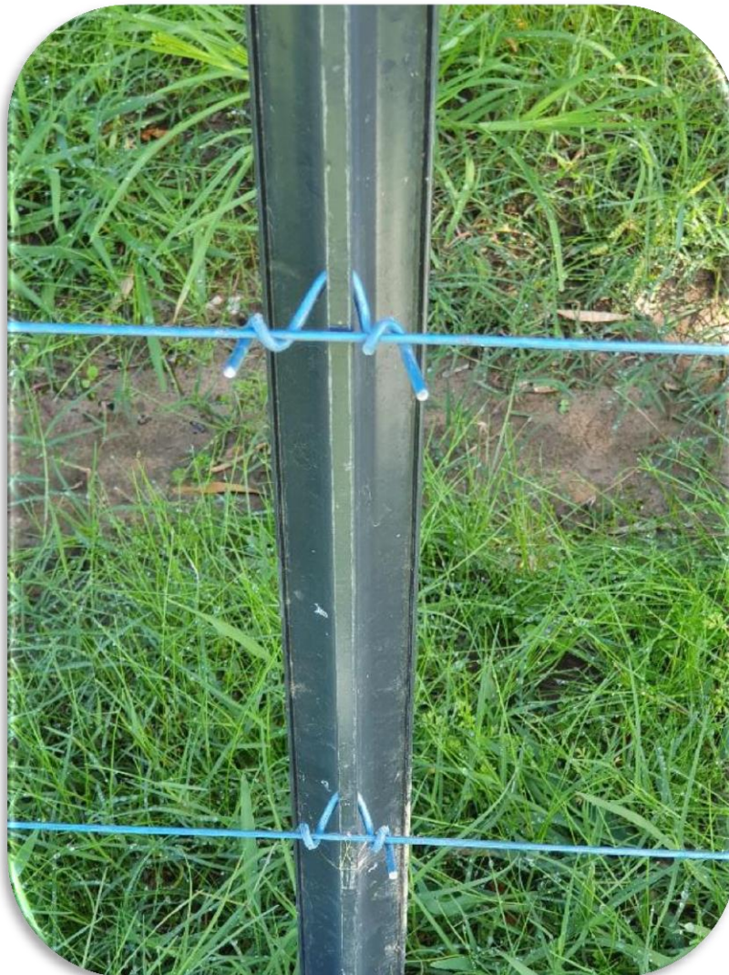
Hot wire (top) and standard wire both attached with standard wire clips.
