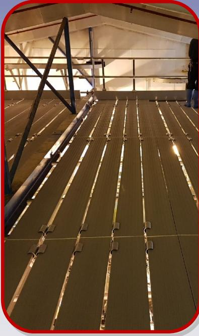
TechBoard polymer based planks present an ideal solution for maintenance in **hygiene sensitive areas** such as dairies. In an environment where the client has banned the use of timber based products the TechBoard integrates perfectly with tube and clip.
