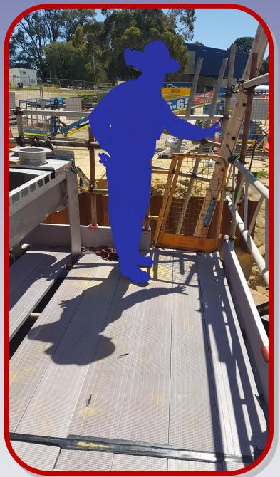
TechBoard being utilised in a tube and clip project for **sandy and often flooded areas** at a waste-water treatment plant upgrade.
